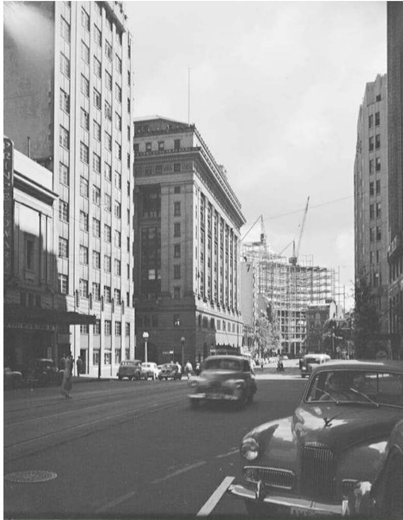
Image 38: Qantas House, Chifley Square, under construction, 1956
