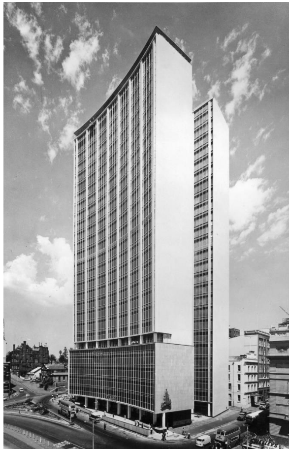
Image 41: AMP Building, facing Circular Quay, mid 1960s ( City of Sydney )
