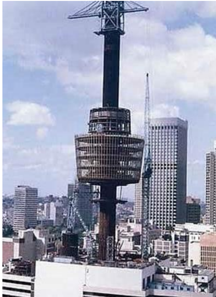
Image 25: Centrepont Tower, Market Street, under construction, late 1970s
