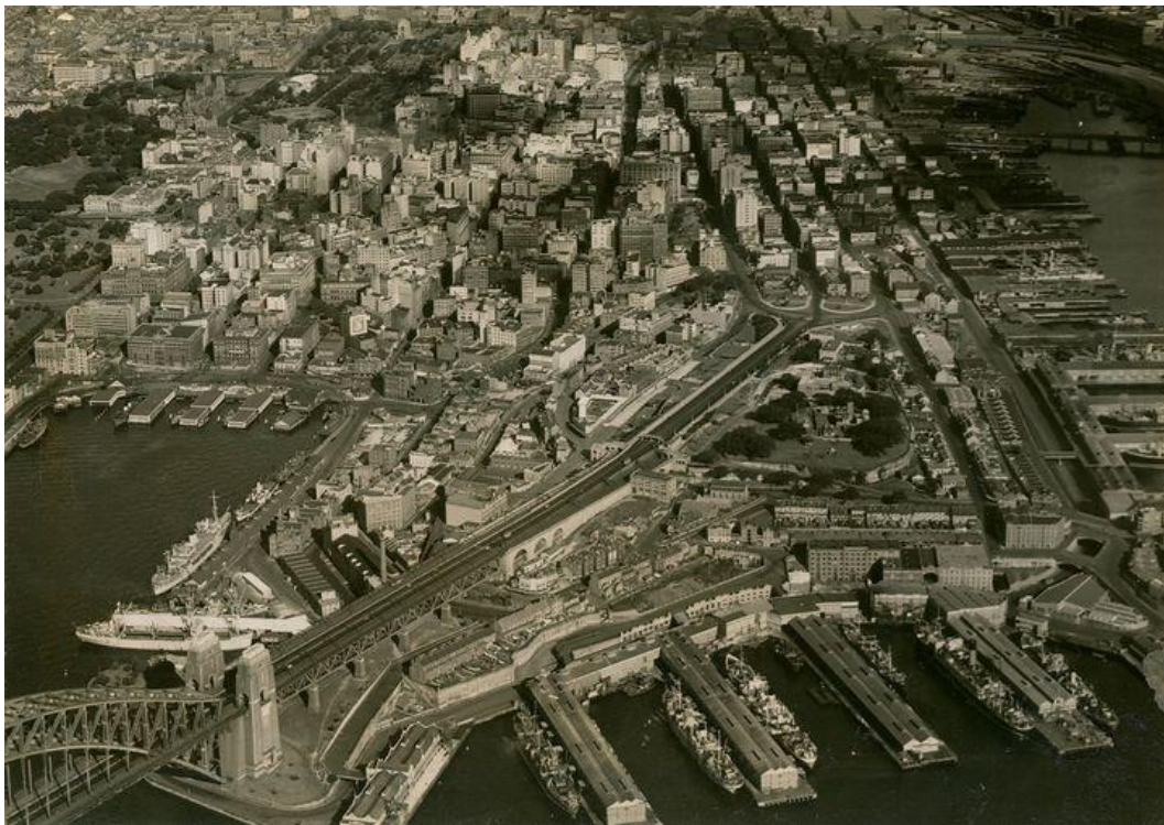
Image 15: Sydney CBD looking from the north, late 1940s ( State Library NSW )
