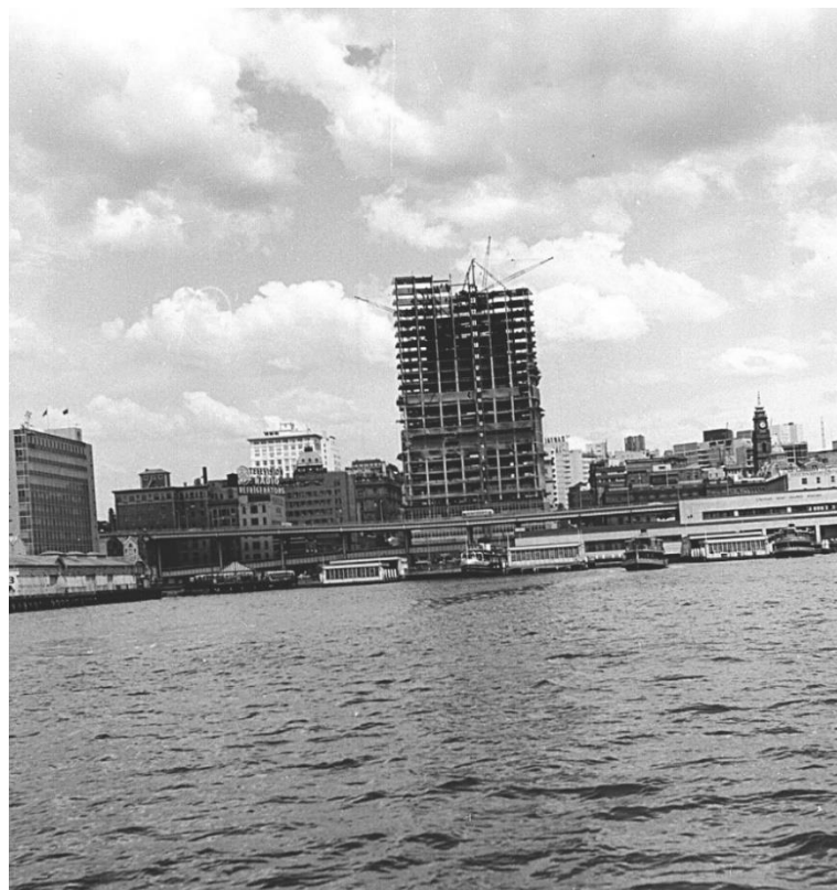
Image 22: AMP Building under construction, Circular Quay, 1960 ( City of Sydney )
