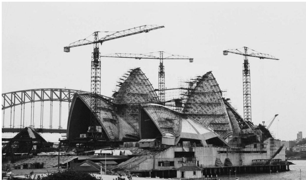
Image 37: Opera House under construction, 1965 ( City of Sydney )
